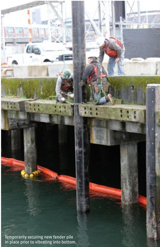
Temporarily securing new fender pile in place prior to vibrating into bottom.
