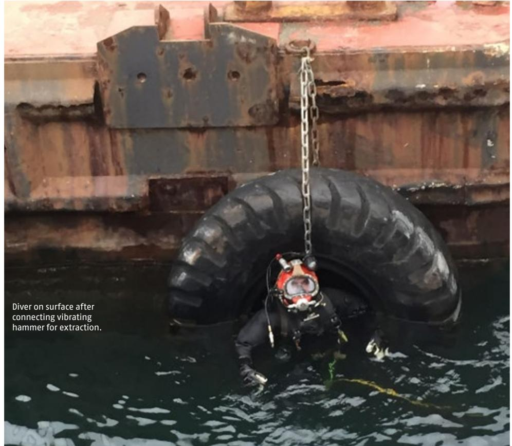
Diver on surface after connecting vibrating hammer for extraction.
